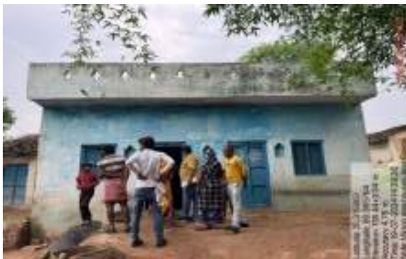
Pic 29: Mining Area houses, Jarur, Banda
